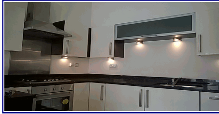
kitchen bulbs replaced
